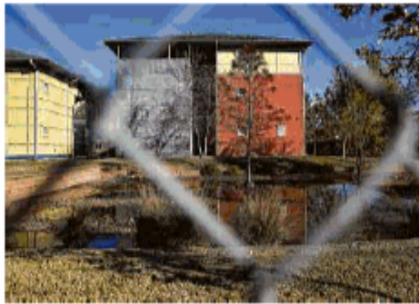
The stormwater infrastructure is designed to minimize the downstream impacts of development.
